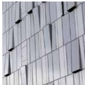
Dominique Perrault Architectes, Paris, (FR) "Onix" office building, Lille, (FR)
