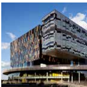
Adjaye Associates, London, (UK) School of Management, Moscow (RU)
