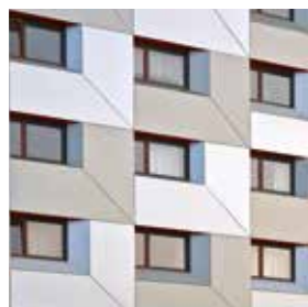
Zimmermann Architectural Cooperative (DE) Student Residence, Dresden, (DE)
